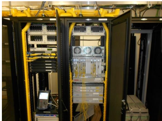
POI Network Equipment (2 of 3)
