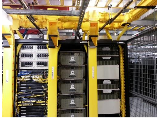
POI Network Equipment (1 of 3)
