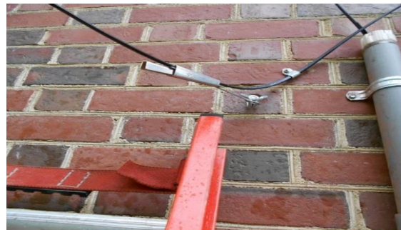
Fiber Optic Drop Cable Connecting to CAI Building
